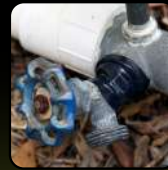
Repairs loose or leaky plumbing
