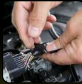
Repairs/insulates electrical wires
